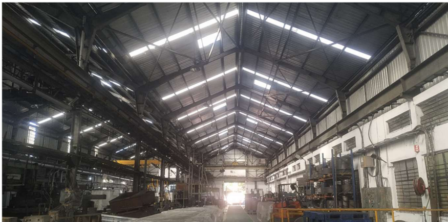
Fig. Adjusted roofing for better lighting
